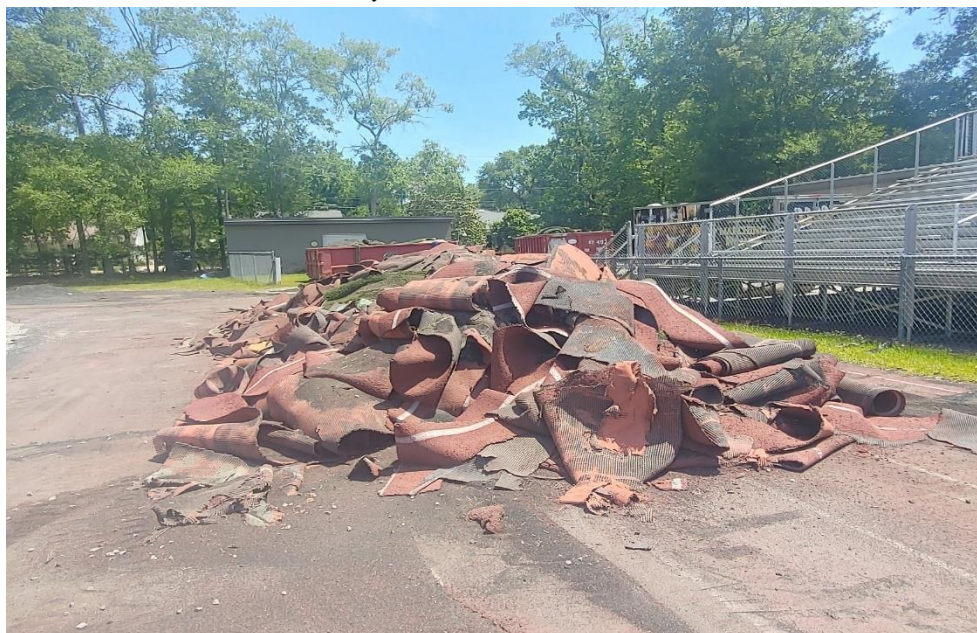
Below: Track remnants ready to be removed.
