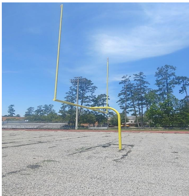
Left: Football uprights in a field of limestone await the new turf.
