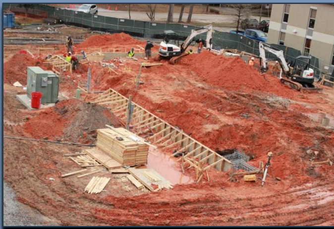
Construction is in full swing.
