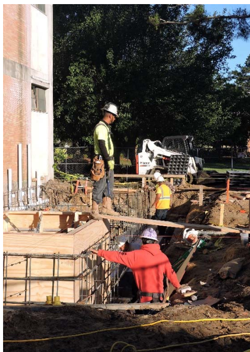
Workers build forms for new restrooms and elevator for Benilde Hall.
