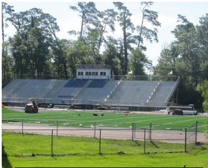
Turf field warranty replacement job nears completion.
