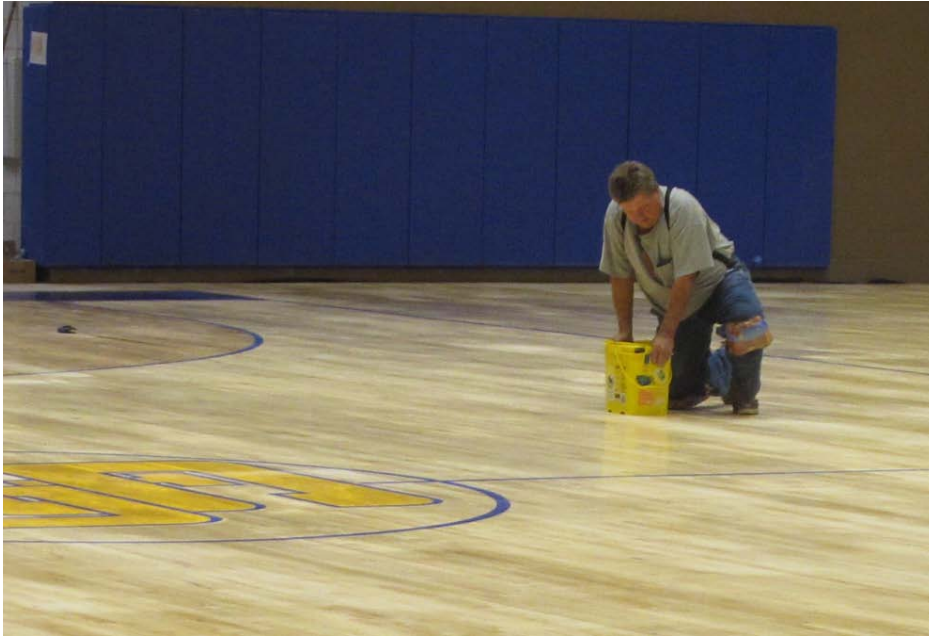
New gym floor nears completion!
