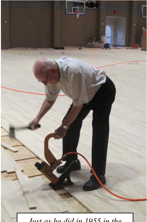
Just as he did in 1955 in the current gym, Brother Alfred helped install floor in the new gym last week – which is rapidly nearing completion.
