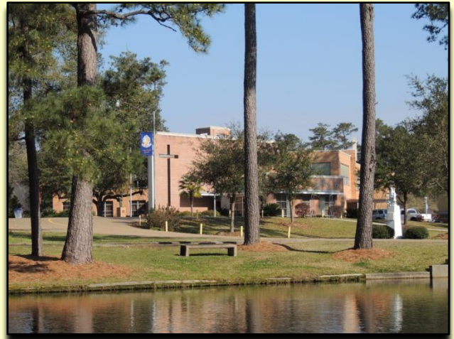
Main School Building today
