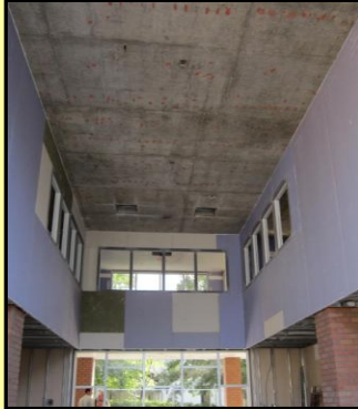
Inside La Salle Hall foyer looking toward the Student Center
