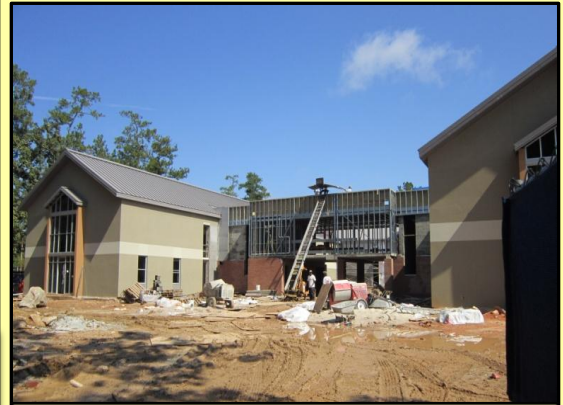
Center wing connecting the two exterior wings
