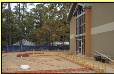
Forming the driveway
